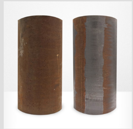
Corrosion Removal on Steel Cylinder
